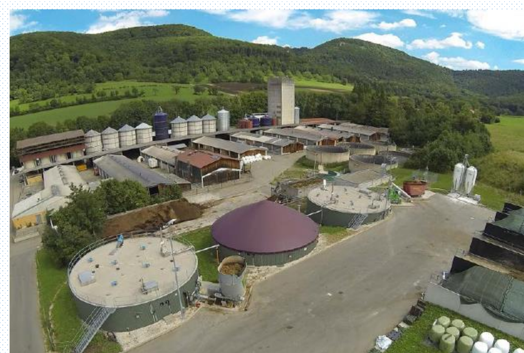
Figure 1. Research biogas plant "Unterer Lindenhof"- Universität Hohenheim
